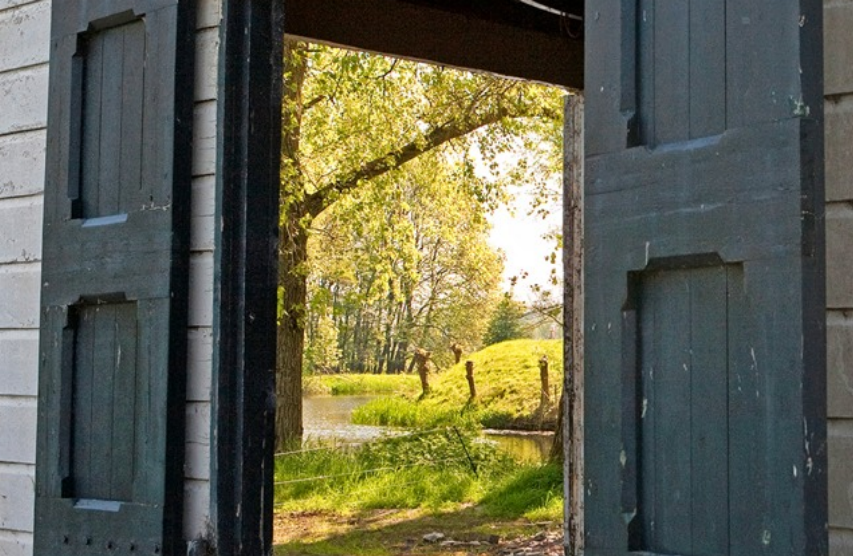
Storage shed at Fort near Nigtevecht.
