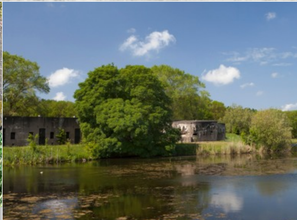
The wet moat of Fort North of Spaarndam.
